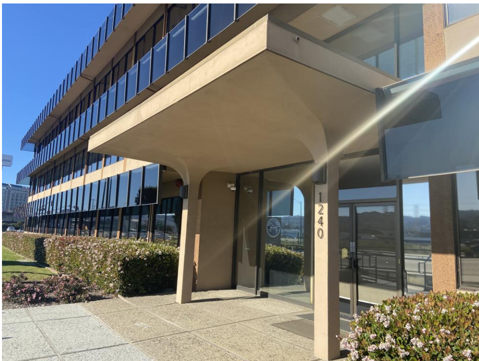
Photograph 4. Main entrance, facing northwest.
