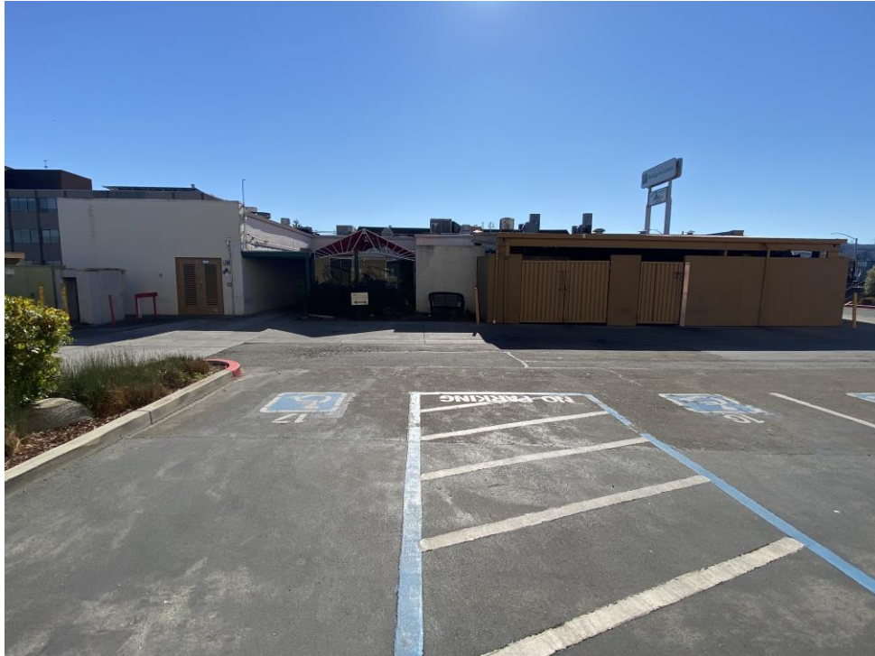
Photograph 3. North (rear) elevation; facing south
