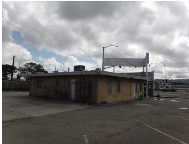
Rear (north) façade, looking south.
