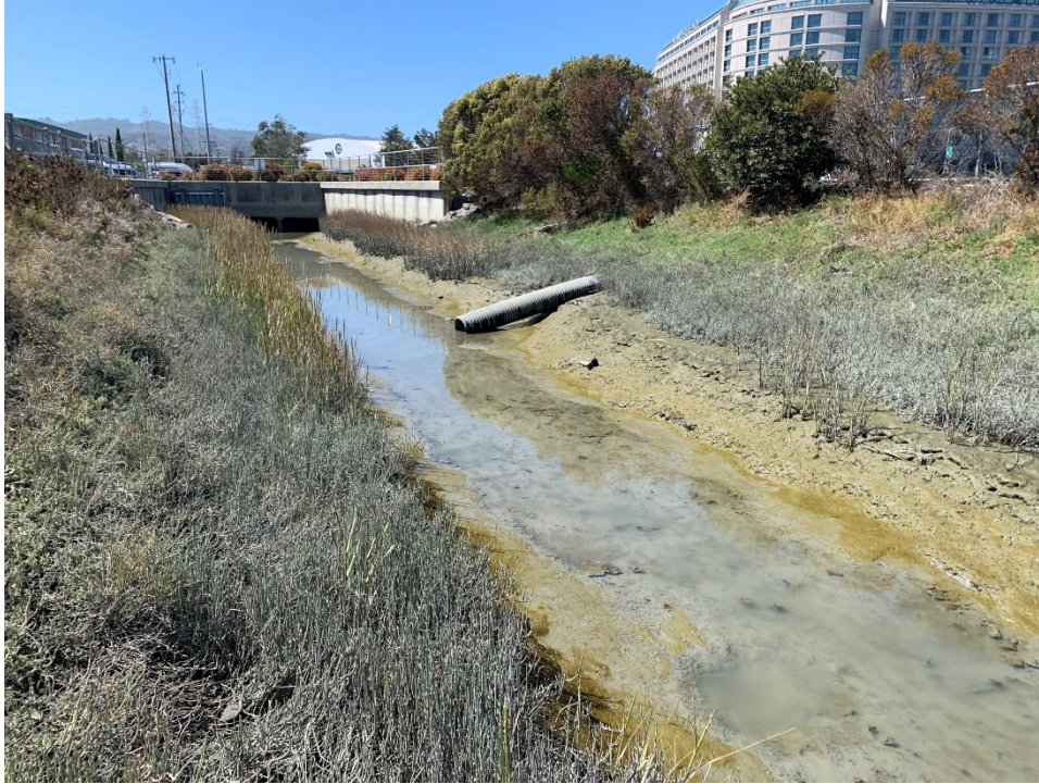
Photo 5. Existing stormwater outfall (to be replaced) near the upper end of the on-site reach of Easton Creek, looking west at low tide.
