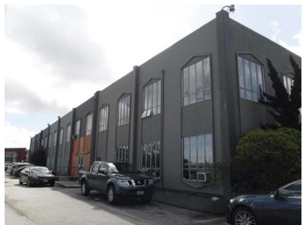
Northeast façade, looking south.
