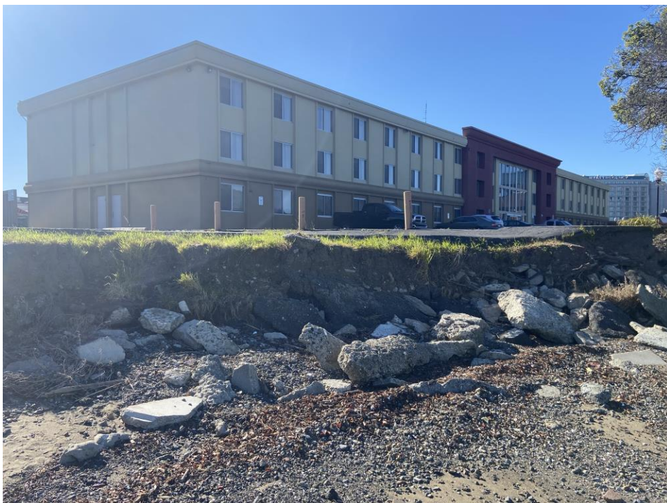
Photograph 4. North and east elevations, view southwest.
