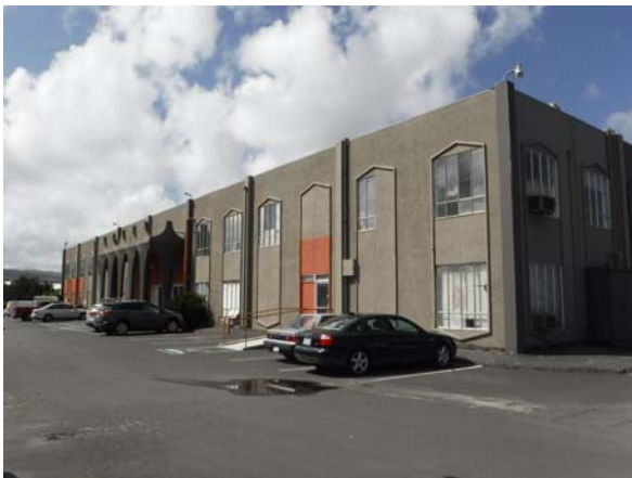
Southeast façade, looking west.
