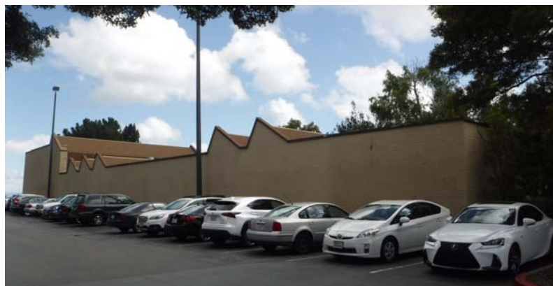
Northwest façade, looking east.
