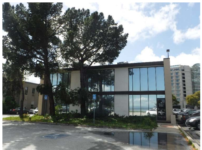
North end of southeast façade, looking west.
