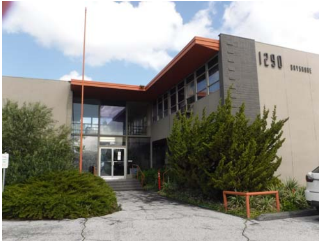
Primary entry, looking northeast.
