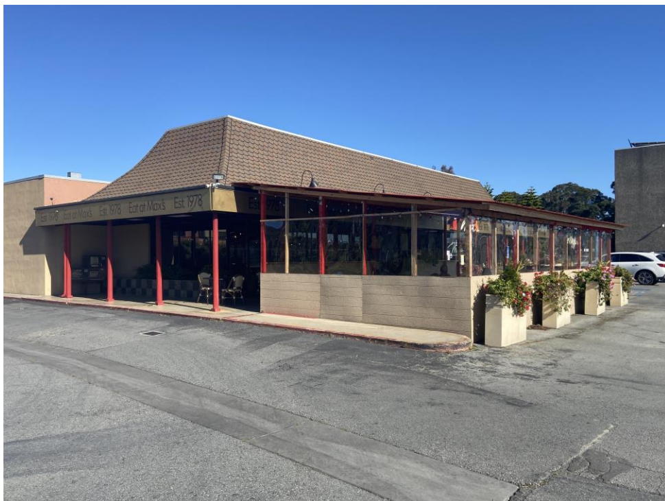
Photograph 4. South and west elevations, view northeast.
