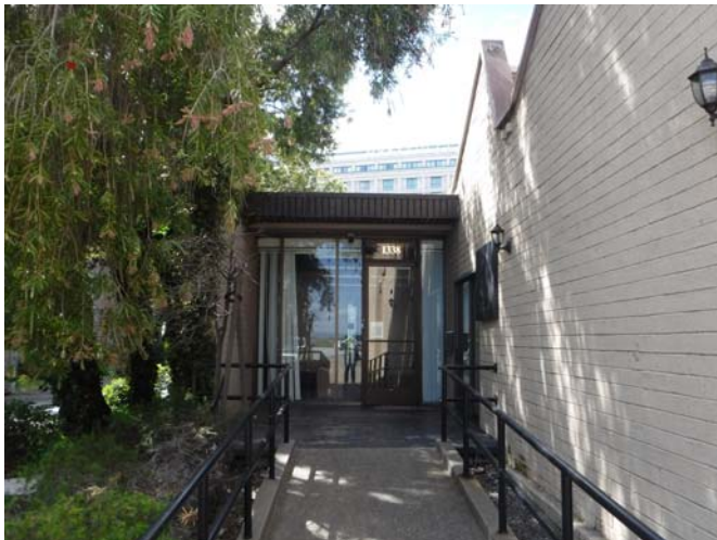
South end of southeast façade, looking west.
