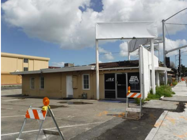
West façade, looking east.
