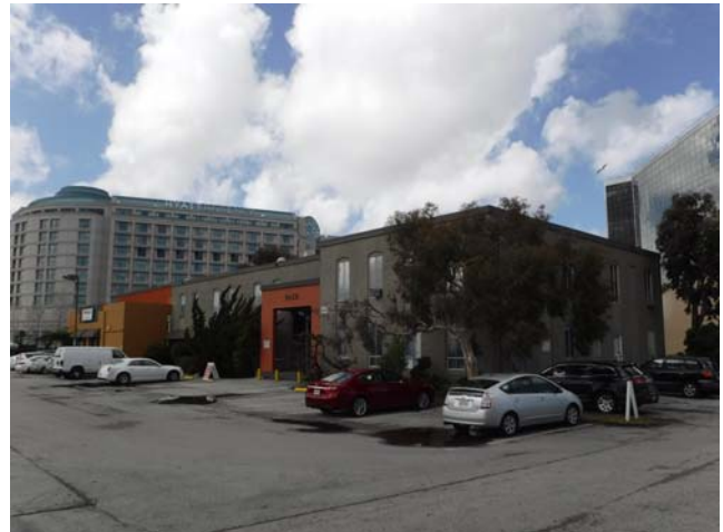
Southeast and northeast façades, looking north.
