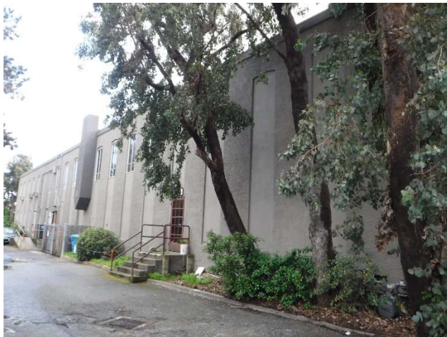
Northwest façade, looking east.
