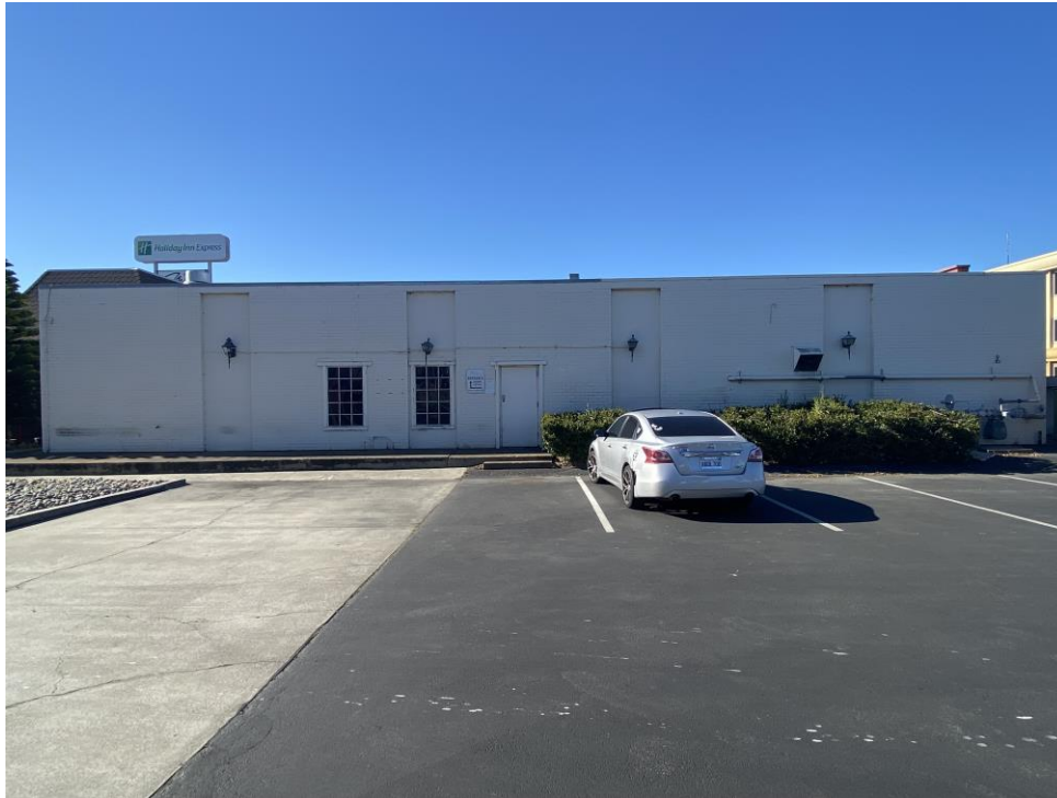
Photograph 2. East elevation, facing west.
