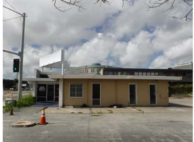
East façade, looking west.
