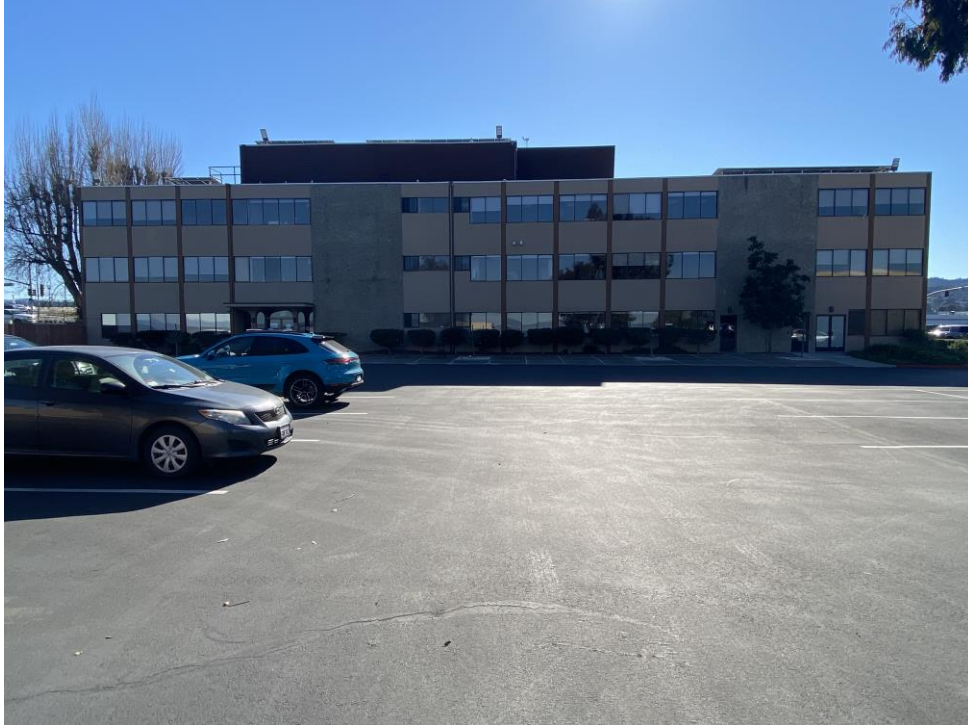
Photograph 3. North elevation; facing south
